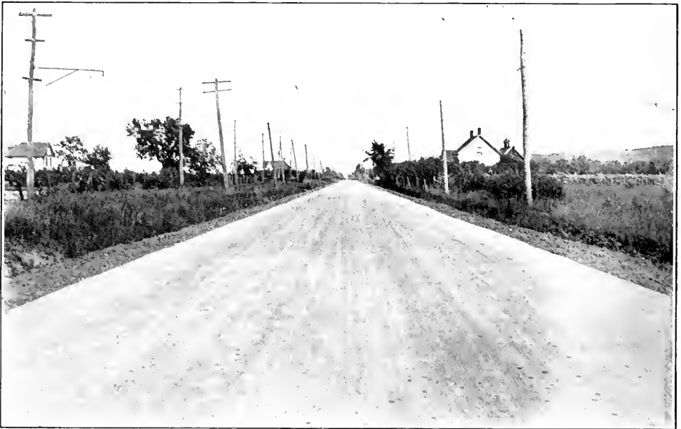
HAMILTON-QUEENSTON PROVINCIAL HIGHWAY Asphaltic concrete surface, east of Stoney Creek.
